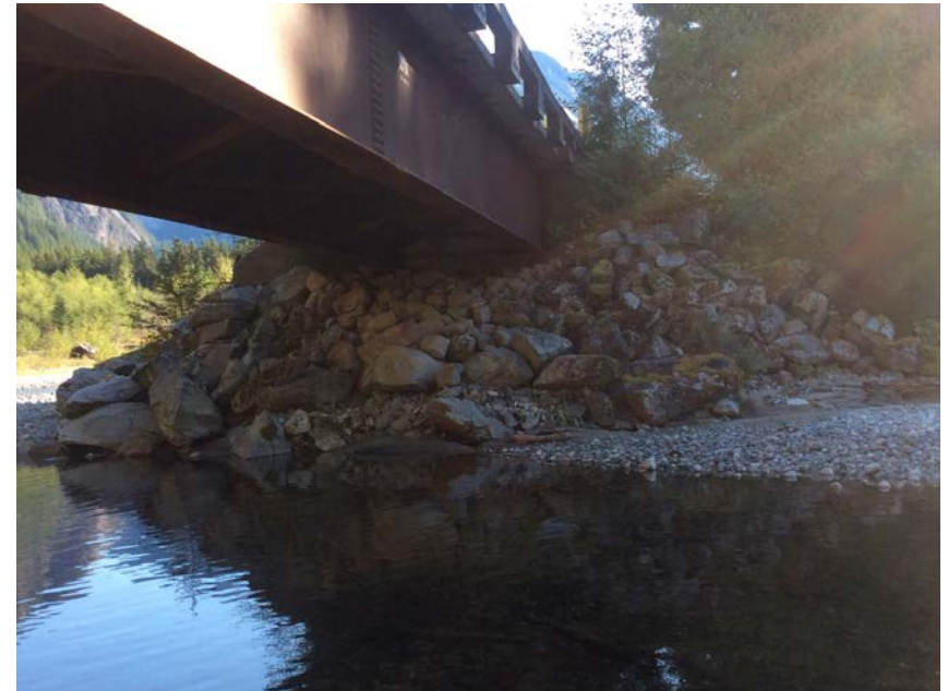
Left Bank Abutment when facing downstream
