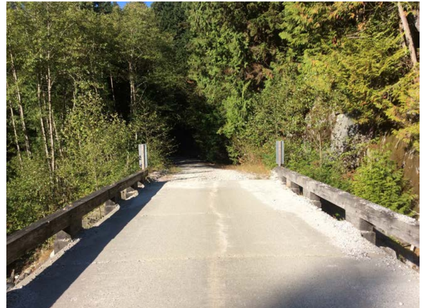
Right approach viewed from bridge
