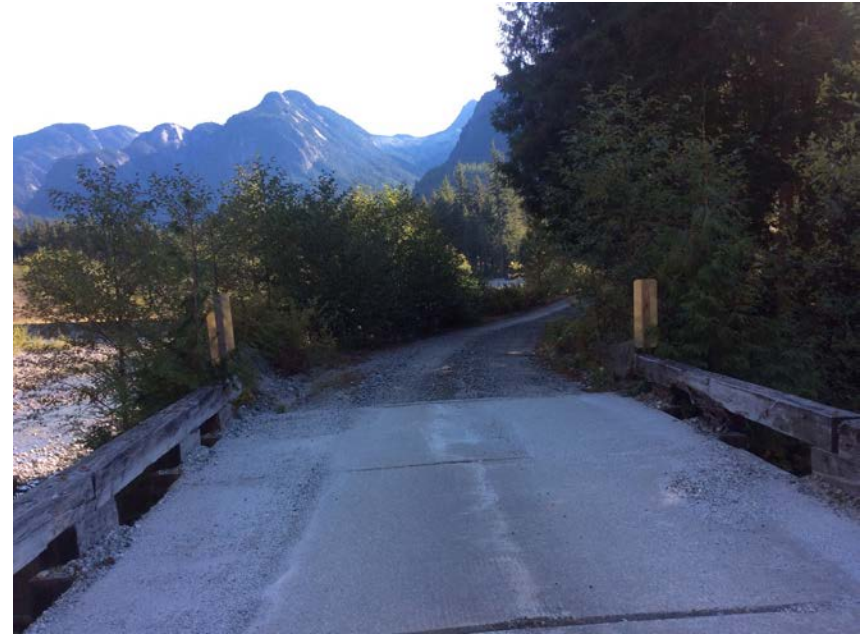
Left approach viewed from bridge
